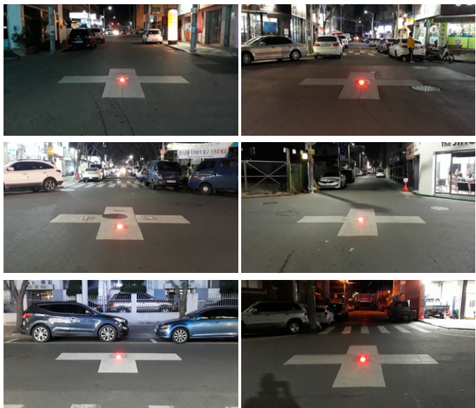
For the Approach of a vehicle blinking red LED
