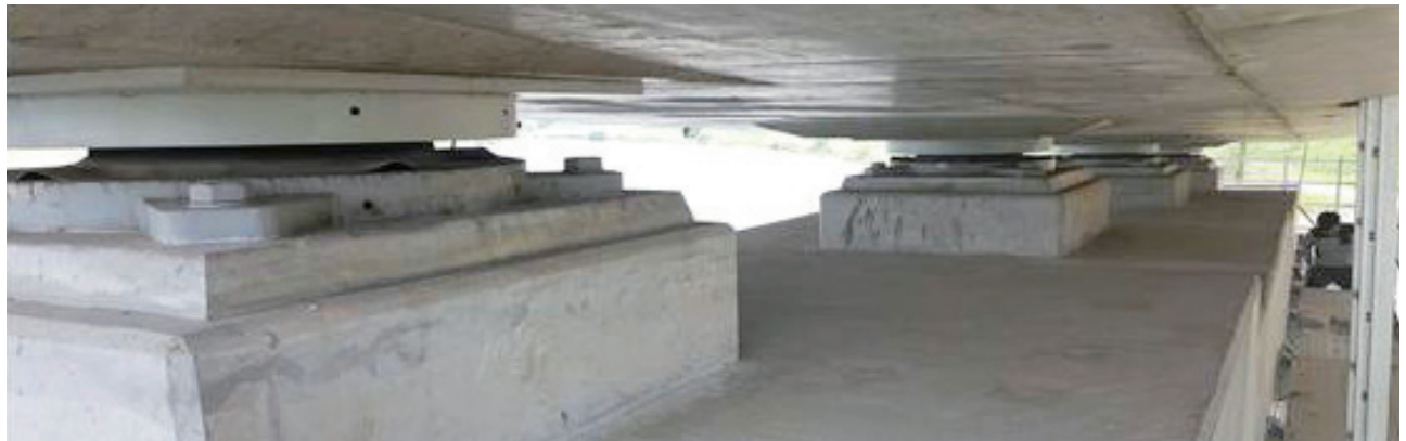
Friction isolation pendulum - Korea expressway corporation
